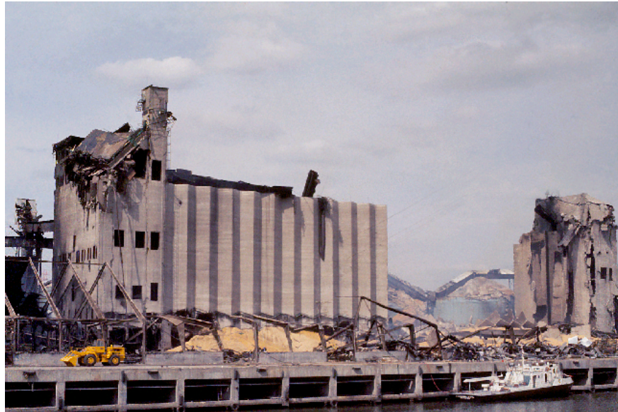
Grain Dust Explosion in Houston, TX 1976
