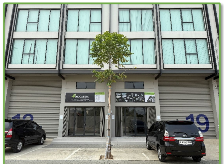
4B Indonesia warehouse & offices
