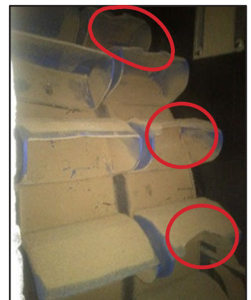
Broken Elevator Buckets
